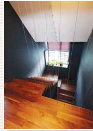
**STAIRWAY (top left)** Black is used on the walls here for dramatic effect while subtly connecting the first and second storeys. To maintain the open concept of the upper level, the designers removed the handrails and replaced them with steel cable. This acts as a safety barrier and allows for the free movement of air and light.
